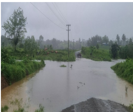
Figure 12e: Vatuwaqa Crossing, Naitasiri underwater on the 26 th . Source: FBC News.
