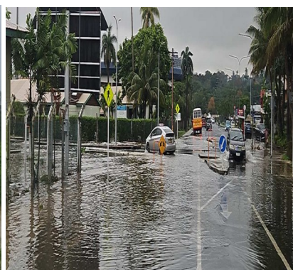
Figure 12f: Surface flooding in Grantham Road on the 26 th . Source: Fiji Roads Authority.
